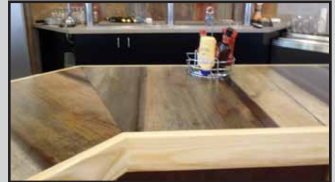
Close-up of Bar Top -- Barnwood Inset, Ash Trim, Epoxy Top
